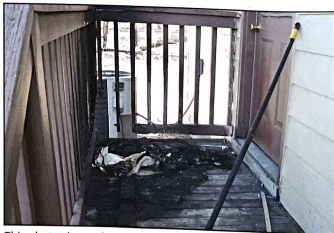
This photo shows damage to a wooden deck from embers.
